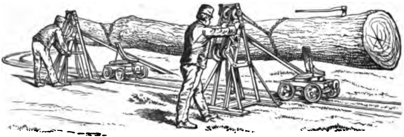
Fig. 219.—Windlass for lading.
